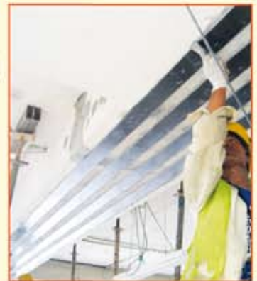
- CFRP Strengthening
