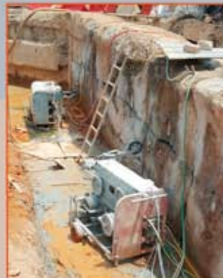
- Diamond Saw Cutting
