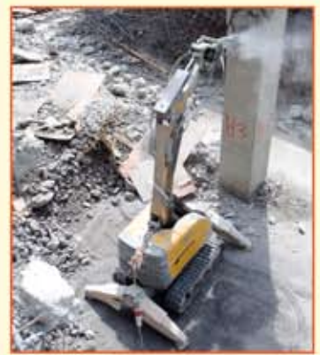
- Brokks Robotic Hacking
